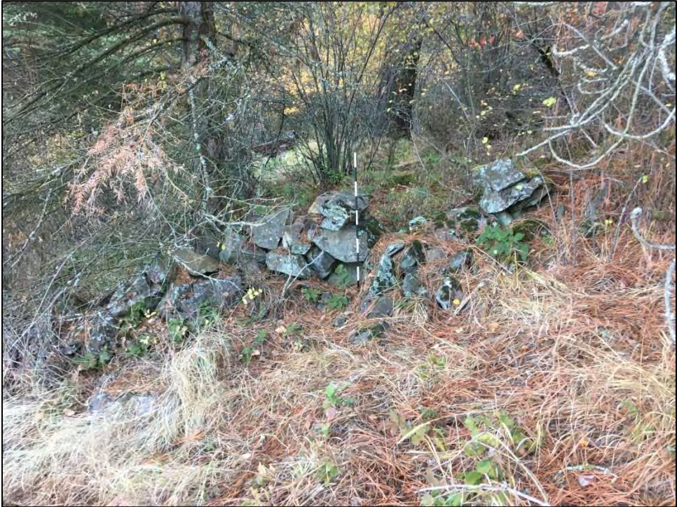
Figure 4. Wall profile near center of wall with game trail opening; view north.
