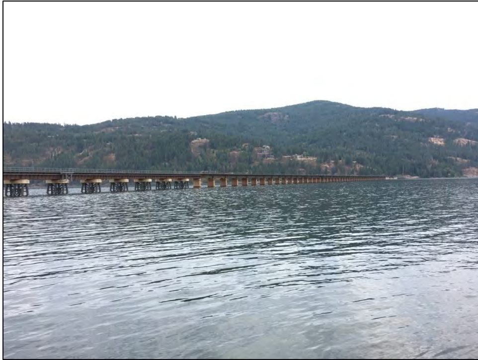
Figure 30. BNSF Bridge 3.9, West Elevation
