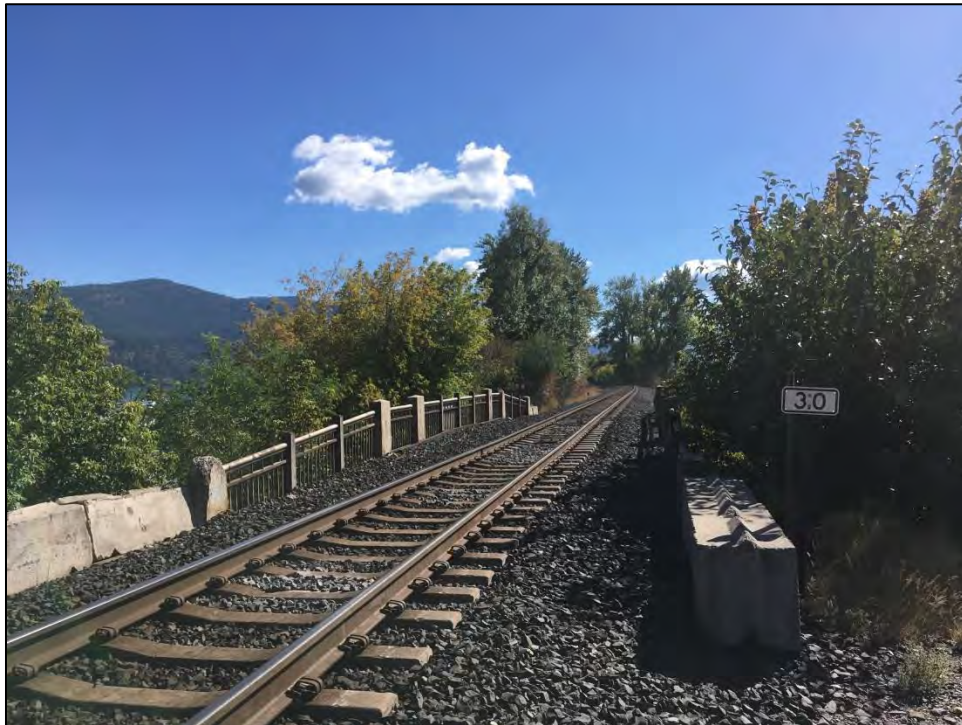
Figure 29. BNSF Bridge 3.1 Railing; View South
