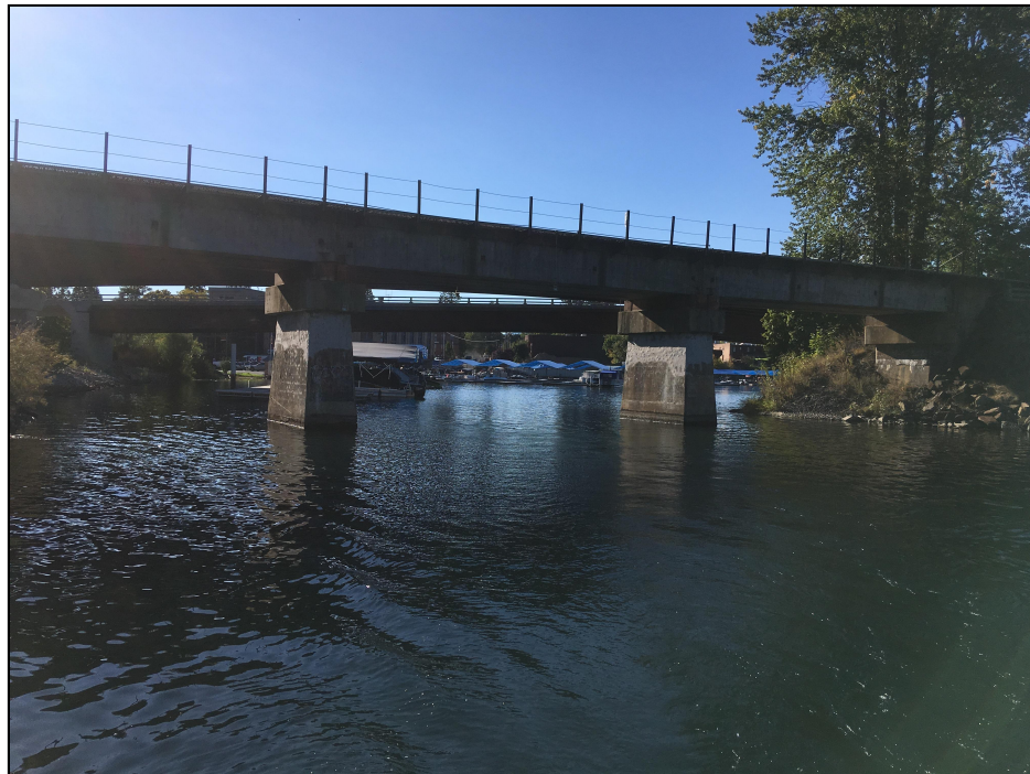
Bridge 3.1, East Elevation
